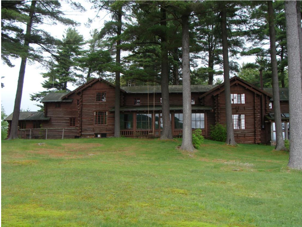
Debar Lodge, south side
